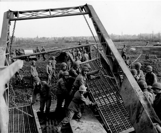
With the assistance of the A-frame from a Brockway truck, Engineers wrestle two treadways into position.
