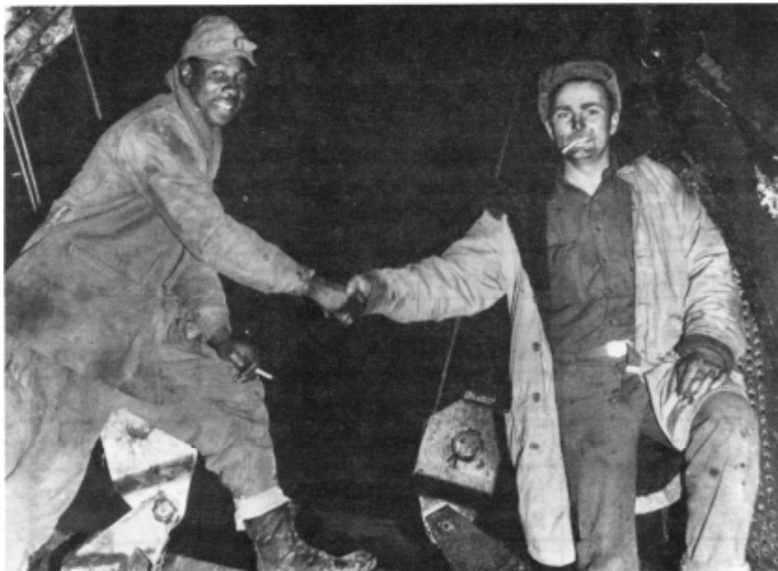
The meeting of the bulldozers at Beaver Creek, Yukon Territory, 25 October 1942 (left: Corporal Refines Sims, Jr., 97th Engineers; right: Private Alfred Jalufka, 18th Engineers).
