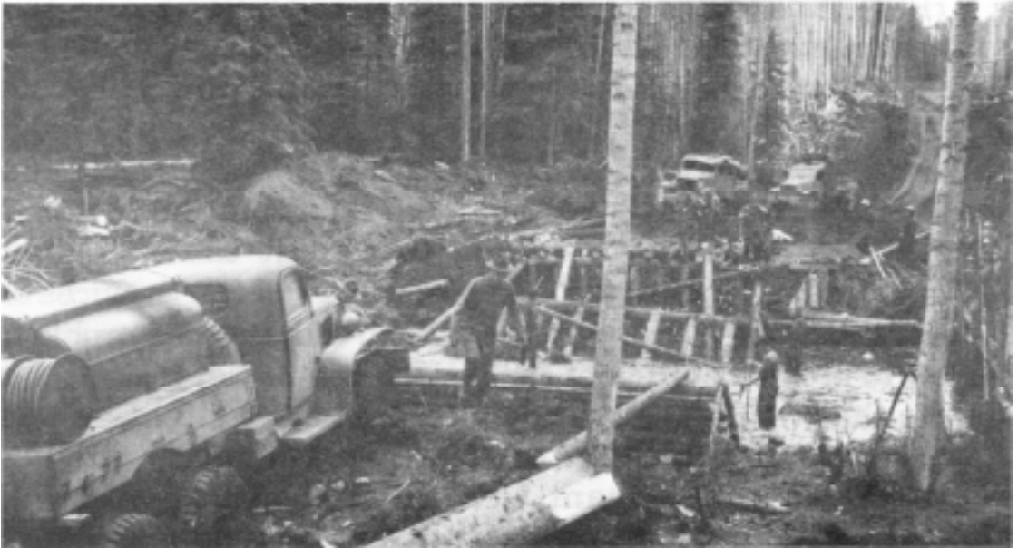
The 18th Engineers build a timber bridge across the Raspberry River north of Whitehorse, Yukon Territory, May 1942.
