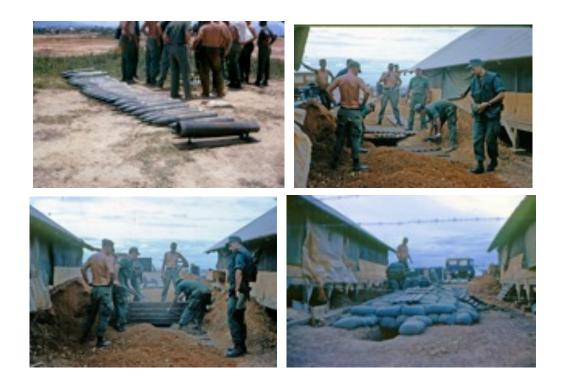
Our days at the airfield were often filled with other surprises, such as the time when a Marine CH-34 came in with a landing gear missing. The following photos show how we saved the day by placing a stack of skids for the bottom of the chopper to rest on as he came in for a landing. Everyone was relieved when the idea worked and allowed the CH-34 to fly again another day.
